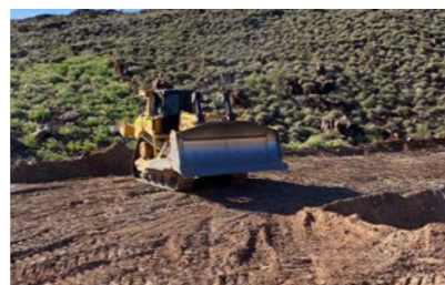
DRILL PAD ACCESS
